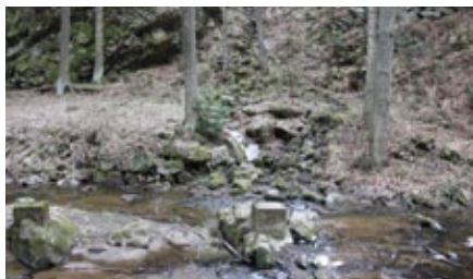
Image 6/ Stone embankment for narrow railway and concrete pillars of the former bridge
