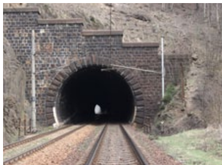
Image 3/ The second tunnel
